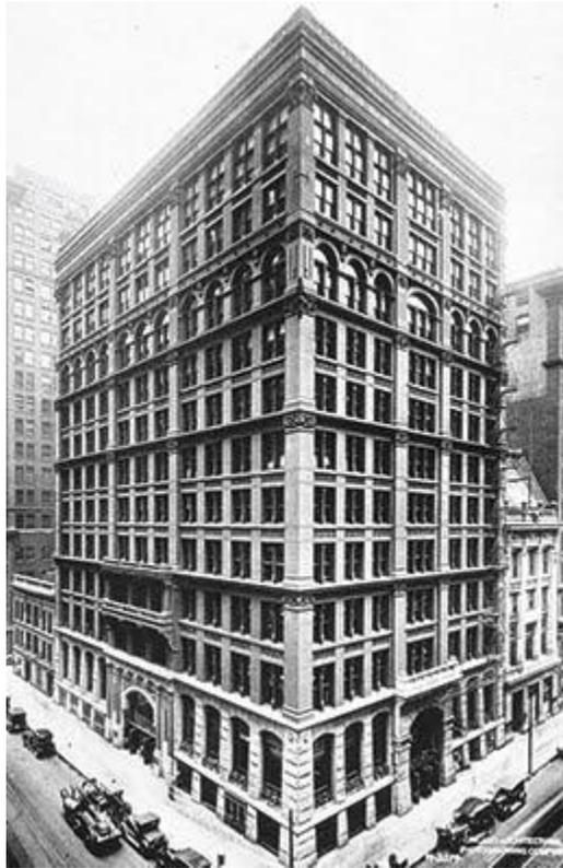
**Figure 4.** While the technology existed to engineer tall buildings, it was not until the invention of the electric elevator in 1889 that skyscrapers began to take over the urban landscape. Shown here is the Home Insurance Building in Chicago, considered the first modern skyscraper.
