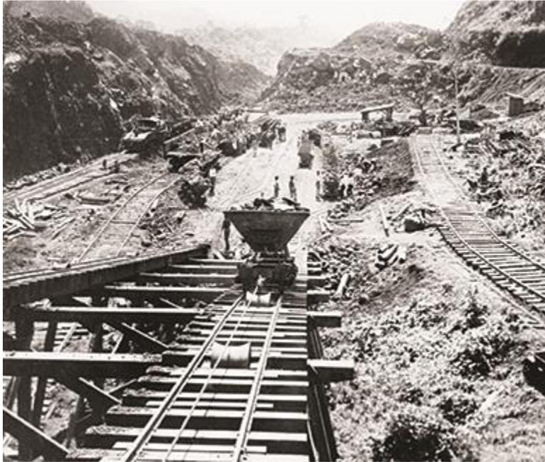
**Figure 2.** Recurring landslides made the excavation of the Culebra Cut one of the most technically challenging elements in the construction of the Panama Canal.
